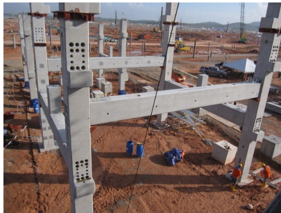
First Overseas Application of SQRIM in a Pipe Rack Structure (Malaysia, 2017)
