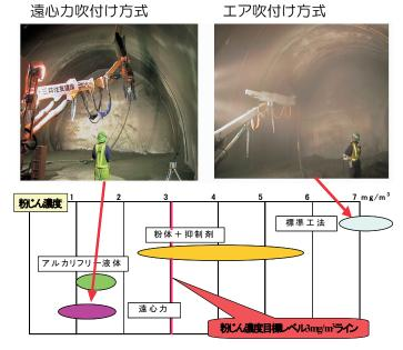
Dust Reduction through Utilization of the Centrifugal Spraying System (Dustless Shotcrete)
