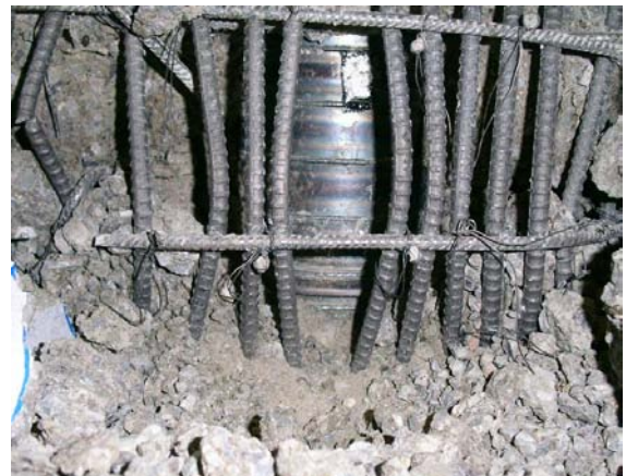
写真-1 鋼管の座屈 (R6-3)
