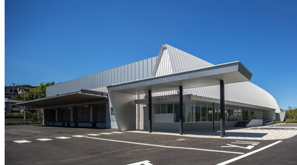
Completed in July 2021
