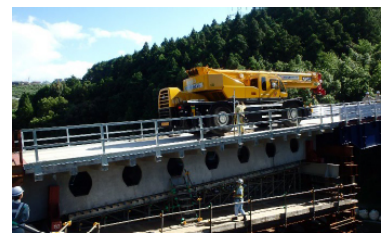
Crane load testing on the demonstration bridge
