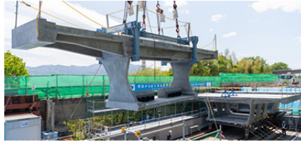
Construction of precast segments
