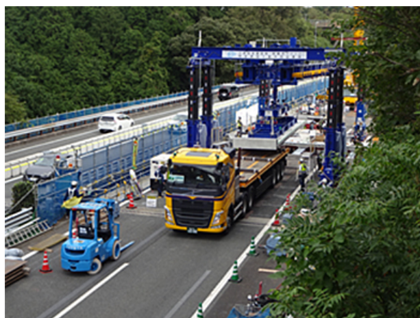
Floor slab replacement work on Tomei Expressway (between Susono Exit and Numazu Exit)
