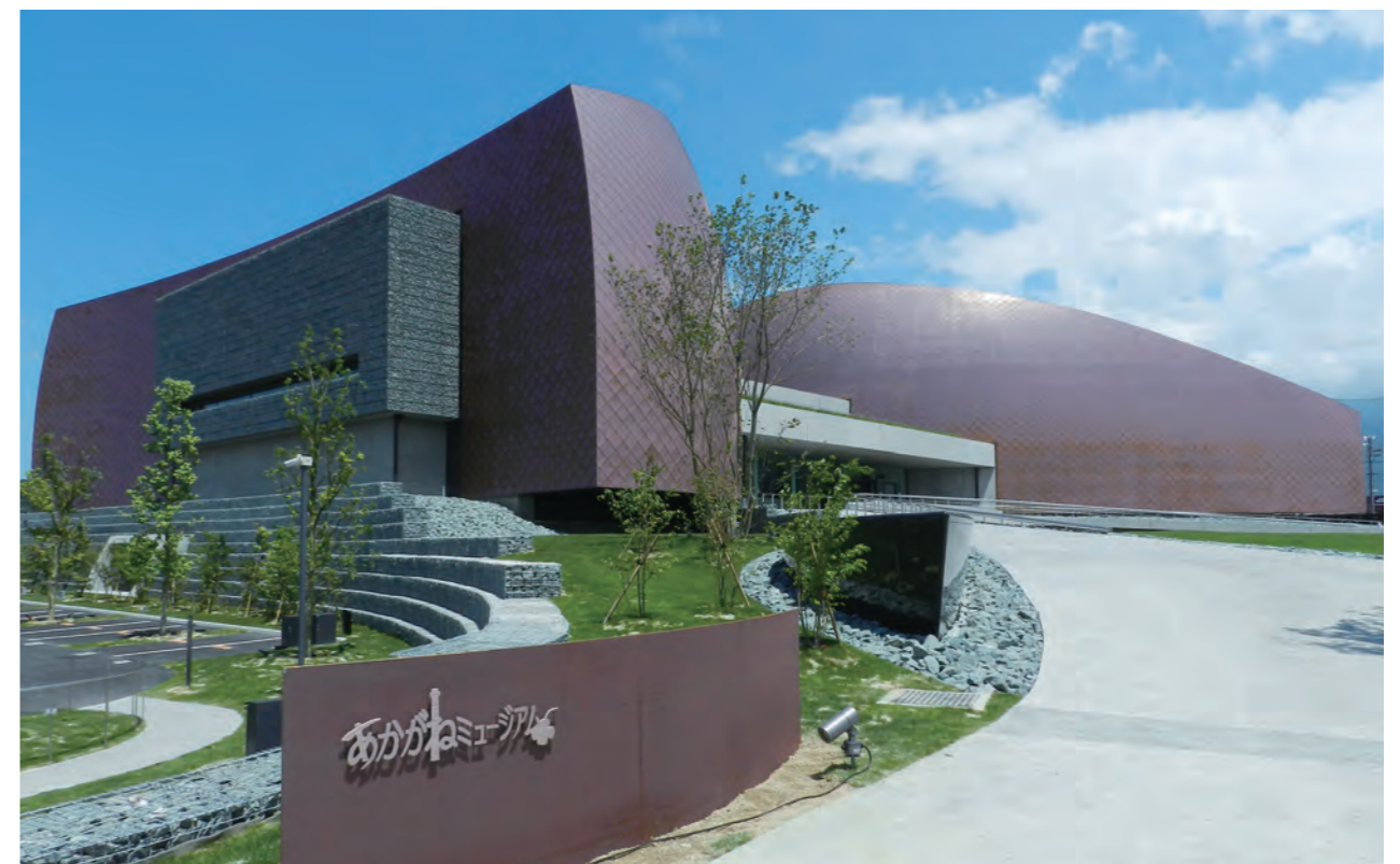
Akagane Museum (Contractee: Niihama City in Ehime Prefecture)
