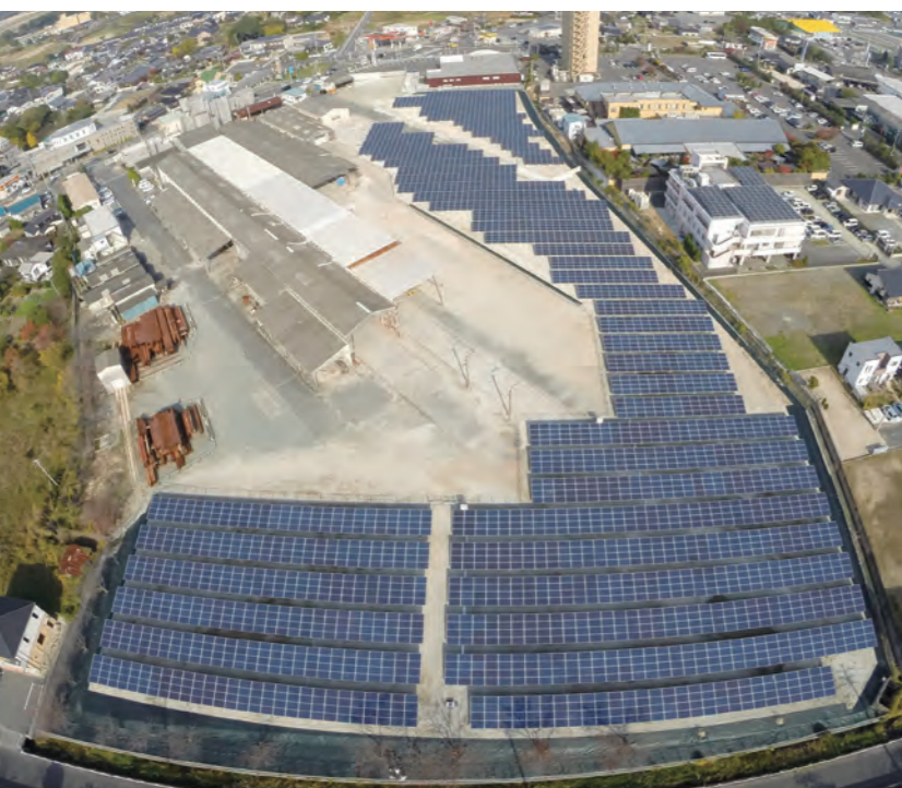
Mitagawa Solar Power Plant
