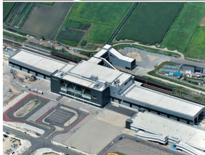
Hokkaido Shinkansen Shin-hakodate-hokuto Station Construction (Contractee: Hokkaido Shinkansen Construction Bureau, Railway Construction Headquarters, Japan Railway Construction, Transport and Technology Agency)
