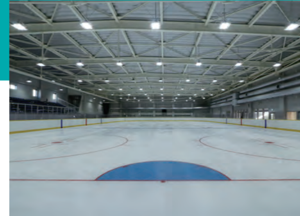
Bank of Yokohama Ice Arena (Kanagawa Skating Rink) (Contractee: Yokohama Sports Association)
