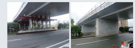
Higashibarū Bridge (Kumamoto Prefecture) emergency restoration underway (left) and after seismic reinforcement (right)
