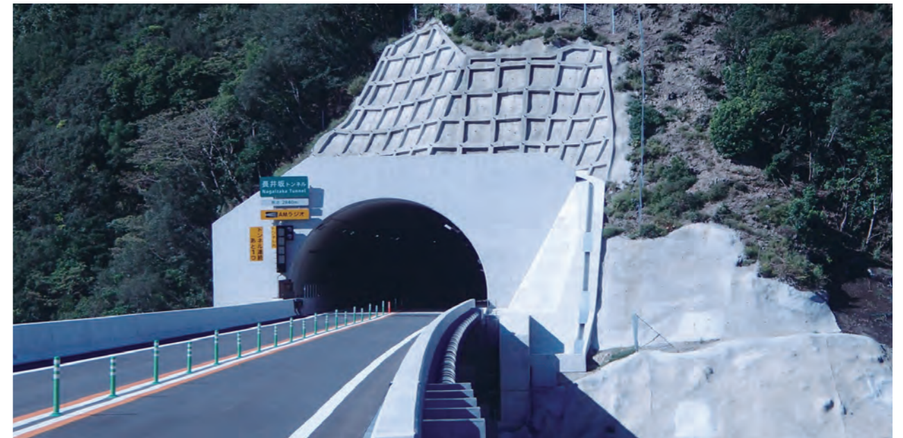
Kinki Expressway Kisei Line Kurotaki Tunnel (Contractee: Ministry of Land, Infrastructure, Transport and Tourism)
