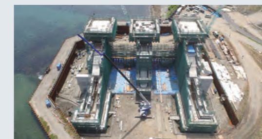
Coast restoration work in Kojirahama area (Iwate Prefecture)
