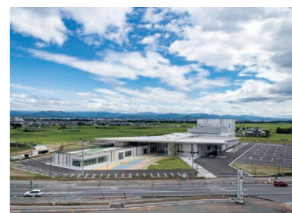
Takizawa City Community Center Development Project (Big Roof Takizawa)
