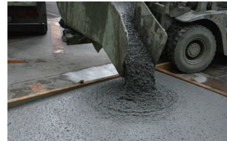
Placing Sustaincrete
