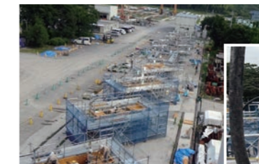
Full view of formwork assembly
