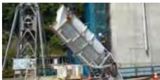
Large-sized bucket for concrete placement
