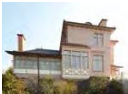
Mid- to large-scale wooden building construction (Shisaka Higurashi House Dismantling and Reconstruction in a Different Place Project)
