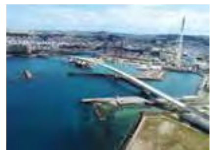
Fiscal 2015 Maki Port Bridge Superstructure (P4-P6) Construction (completed in 2017, contractee: Development Construction Department, Okinawa General Bureau, Cabinet Office)
