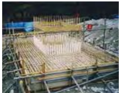
Foundation of tensioning portal using aramid rod for electricity reception
