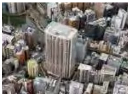
Brillia The Tower Tokyo Yaesu Avenue (completed in 2017; contractees: Tokyo Tatemono Co., Ltd. and Mitsubishi Jisho Residence Co., Ltd.)
