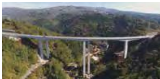
Washimi Bridge overview
