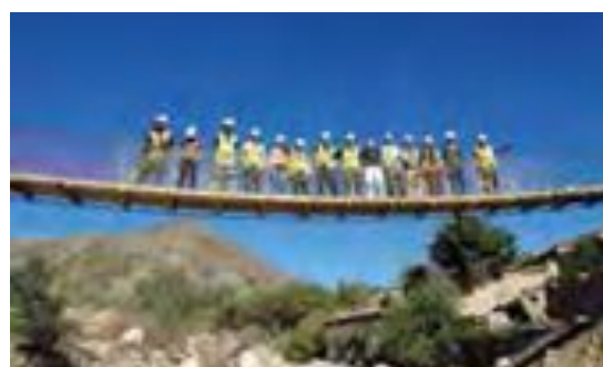
Pedestrian bridge construction project in Bolivia
