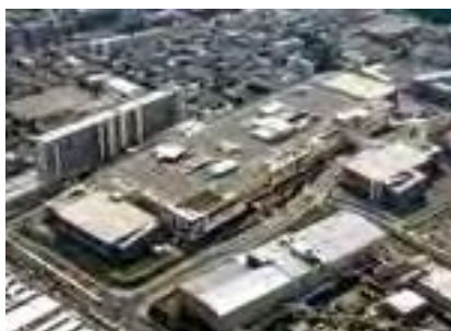
Lalaport Shonan Hiratsuka (completed in 2016; contractee: Hiratsuka Special Purpose Corporation)
