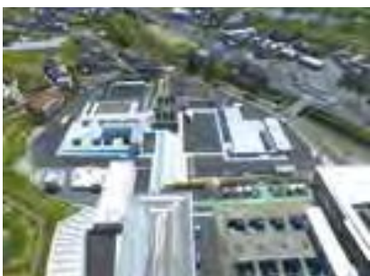
Odanaka Purification Plant Renovation (completed in 2016, contractee: Tsuyama City Waterworks Bureau in Okayama Prefecture)
