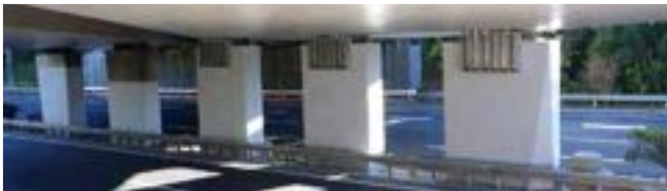
Joban Expressway Hiro-oka Bridge Seismic Reinforcement Project (contractee: East Nippon Expressway Co., Ltd.; received Fiscal 2019 Excellent Project Manager Award)
