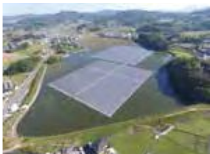
Solar power generation (Hiragioike Floating Solar Power Generation Plant [own business])
