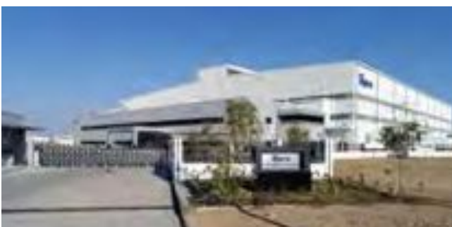
Topre Corporation Gujarat Press Plant Construction (India)
