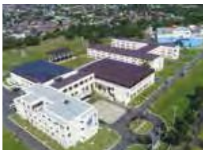
MOL Magsaysay Maritime Academy Construction (completed in 2018; contractee: MOL Magsaysay Maritime Academy, Inc. [Local subsidiary of Mitsui O.S.K. Lines, Ltd.]
