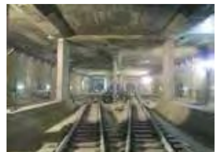
Jakarta MRT Construction Project CP106 Section (completed in 2019; contractee: PT Mass Rapid Transit Jakarta)
