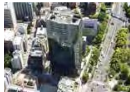
Sumitomo Realty & Development Onarimon Tower (completed in 2018; contractee: Sumitomo Realty & Development Co., Ltd.)
