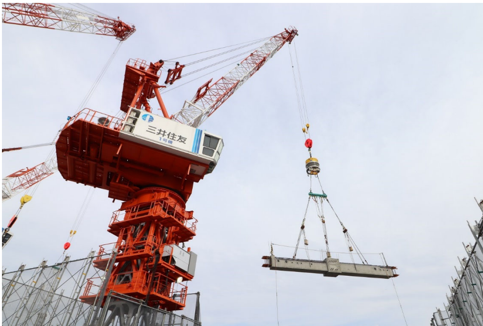
[Tower crane operation support system and Roborigger]
