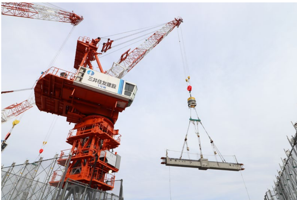
[Tower crane operation support system and Roborigger]
