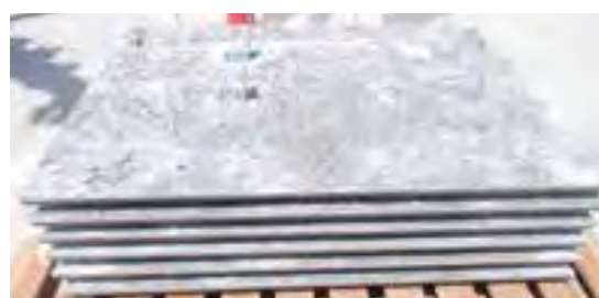
Precast embedded formwork
