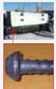
Upper: An application to PCa bridge railing Lower: Enlarged photo of the end of Trunc-head
