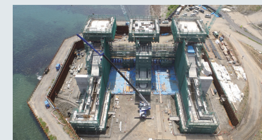
Coast restoration work in Kojirahama area (Iwate Prefecture)
