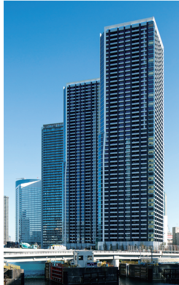
DEUX TOURS CANAL&SPA (Contractee: Sumitomo Realty & Development Co., Ltd.)
