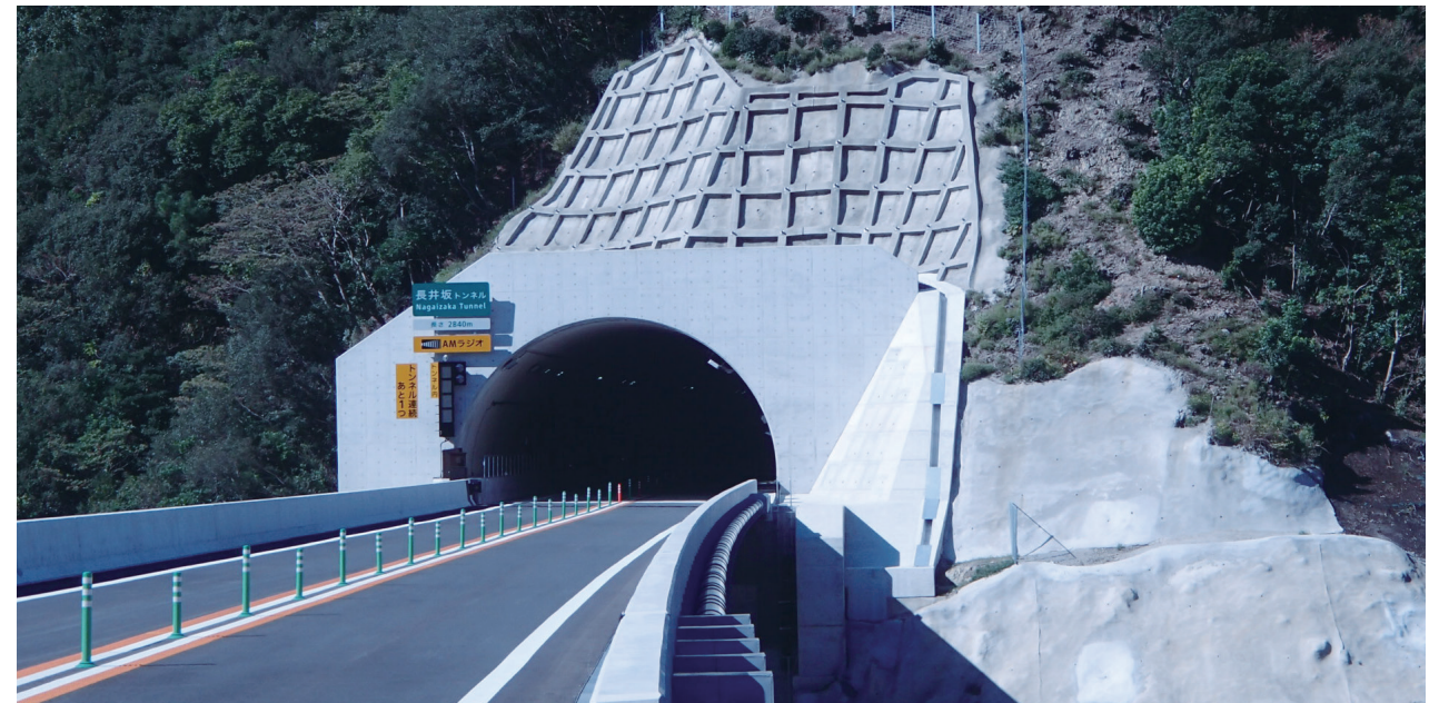
Kinki Expressway Kisei Line Kurosaki Tunnel (Contractee: Ministry of Land, Infrastructure, Transport and Tourism)
