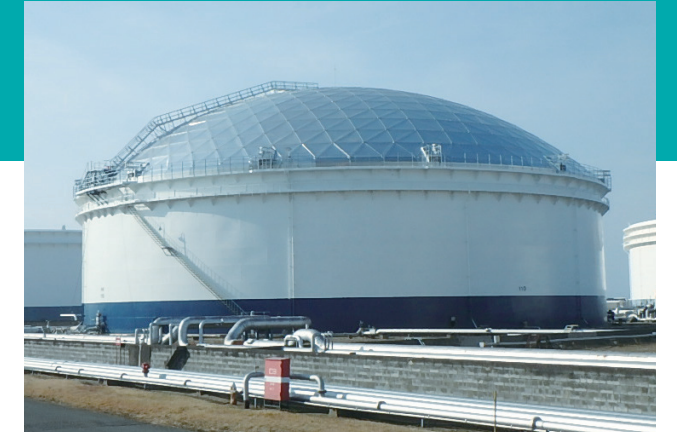
Petroleum product storage ultradome (Contractee: JX Nippon Oil & Energy Corporation)
