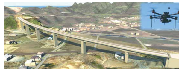
Synthetic view of an automatically created image of bridge and the landscape captured by a drone
