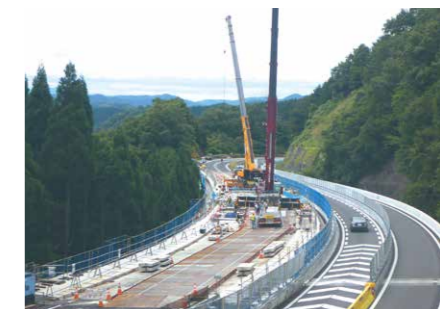
Installing precast PC floor slabs
