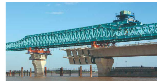
World's largest span-by-span bridge construction (Lach Huyen Bridge, Vietnam)
