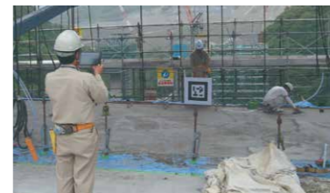
Height management using tablet terminals
