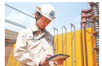
Inspecting reinforcement placement using a tablet computer
