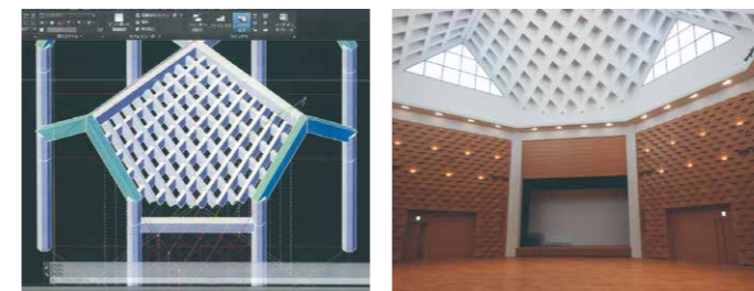
3D modeling data (left) and completed state (right) of Yamazaki Baking Central Laboratory Hall
