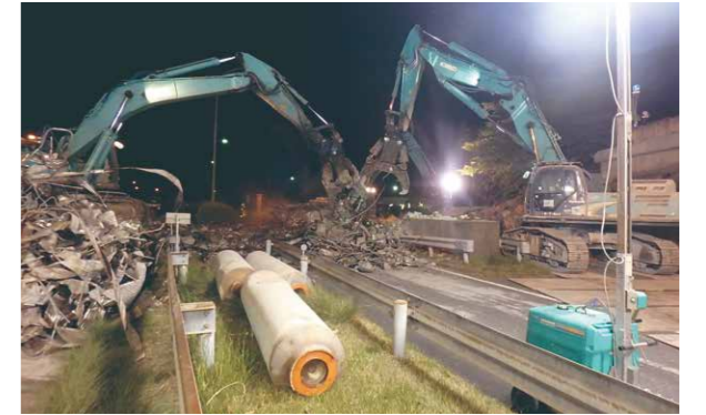
Removing the Furyo Bridge
