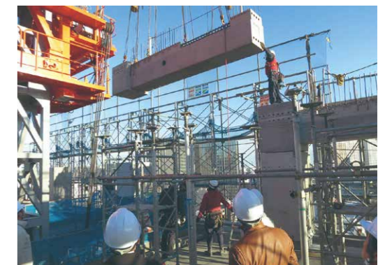
Site visit by the Quality and Functional Housing Committee
