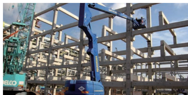
Plant (pipe rack) construction in Malaysia
