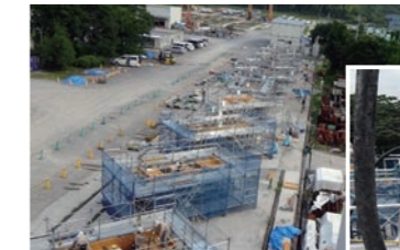
Full view of formwork assembly
