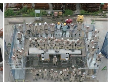
Completed two-girder concrete placement
