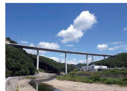
Shin-Meishin Mukogawa Bridge
