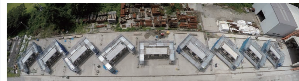
Full view of completed skeleton concrete placement
