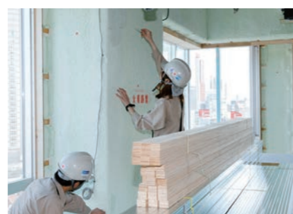
Checking the thickness of spray-applied insulation
