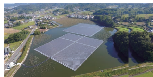
Hiragioike Solar Power Generation Plant (own project in Kagawa Prefecture)
