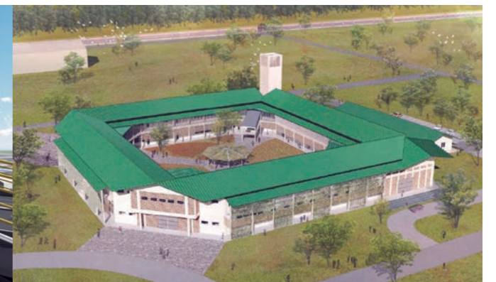
The Project for the Establishment of Research and Training Complex at the Faculty of Agriculture, University of Jaffna (Courtesy of Japan International Cooperation Agency [JICA])
