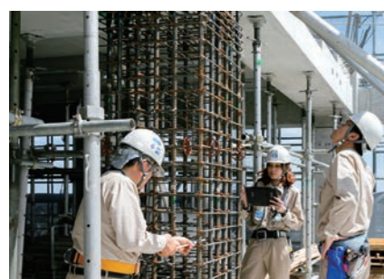
Checking bar arrangement in reinforcement placing
