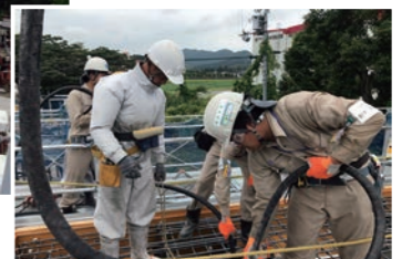
Placing concrete
