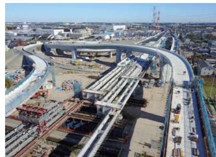
PC superstructure construction adopting precast U-girder segments
