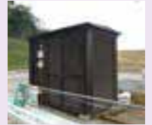
A bio-toilet being installed at a Company site
