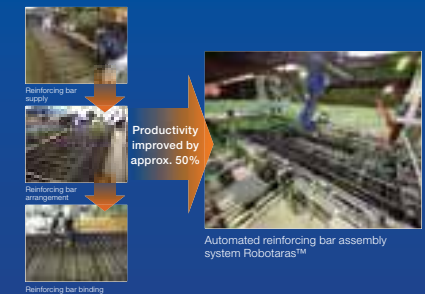
Using robots to automate the arrangement and bundling of reinforcing bars
