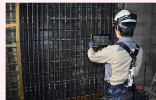
Inspection using Raku Camera ®
