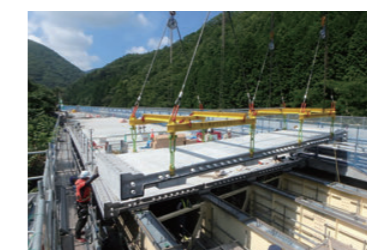
Floor slab replacement for the Tadeno No. 2 Bridge (Outbound)
