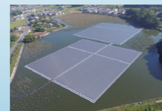
Hiragioike Floating Solar Power Generation Plant
