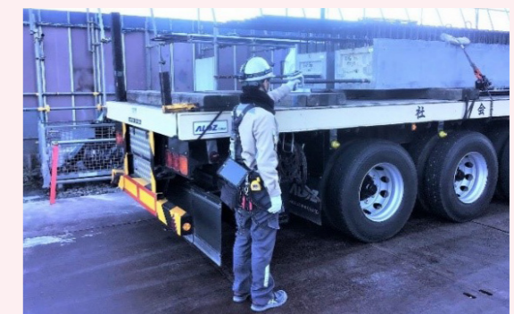
Reading RFID tags upon delivery to site
