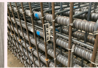
RFID tag-integrated spacer attached to a rebar
