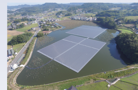
Hiragioike Floating Solar Power Generation Plant
