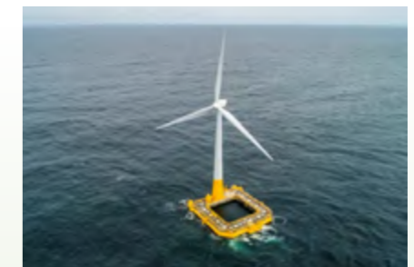
BW Ideol's demonstration unit (Photo credit: BW Ideol / V. Jonchery)
