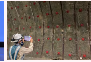
Lock bolt interval measuring system
