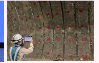
Lock bolt interval measuring system
