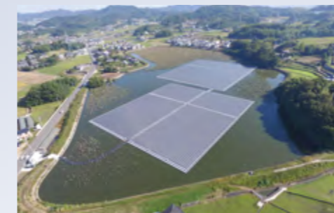
Hiragioike Floating Solar Power Generation Plant
