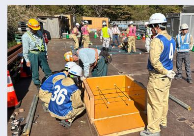
Experience rebar binding work
