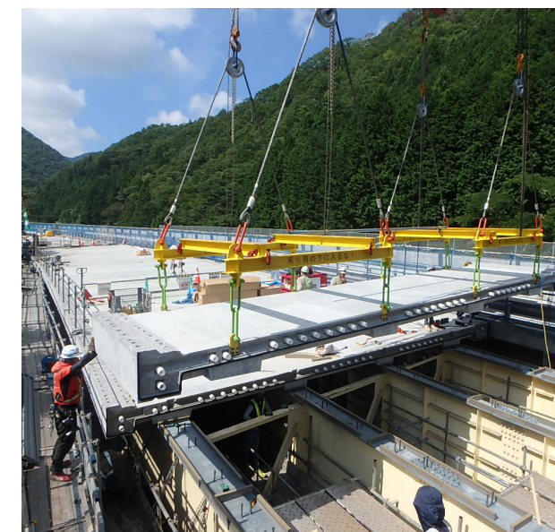
Replacement work of deck slabs on the Second Taden Bridge and three other bridges (Shimane Prefecture)
