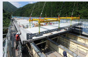
JPCI Award for Outstanding Structures (Renovations Category) Deck slab renewal work of Taden Second Bridge Downstream Line
