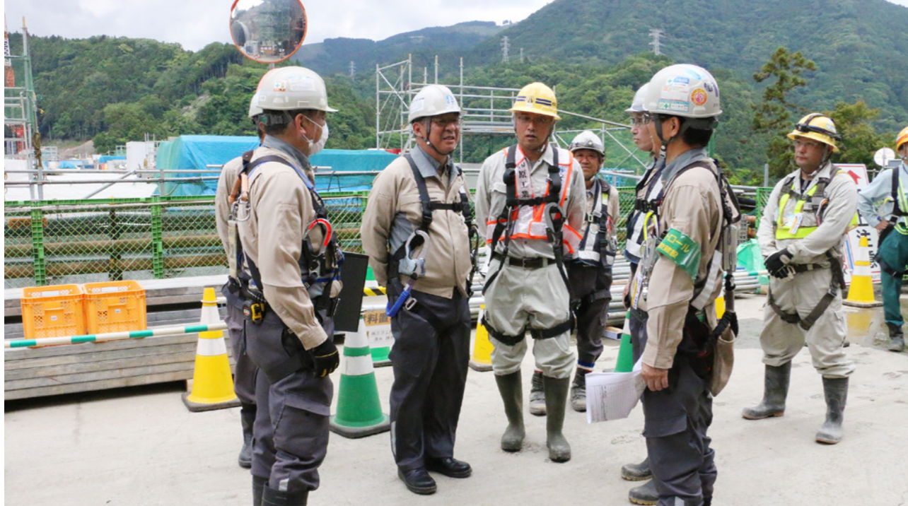
Construction in Yamakita Minasegawa on the Shin-Tomei Expressway
