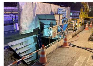
Quick-re-Invert Method (using Messer shield machines)
