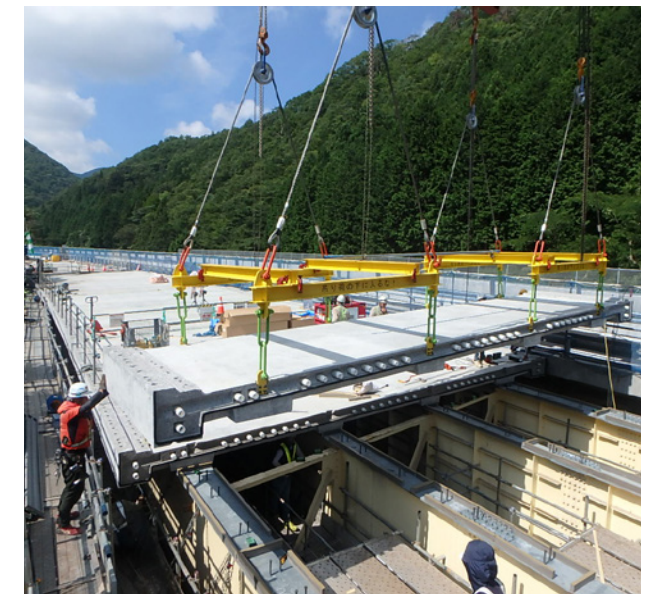
Replacement work of deck slabs on the Second Taden Bridge and three other bridges (Shimane Prefecture)
