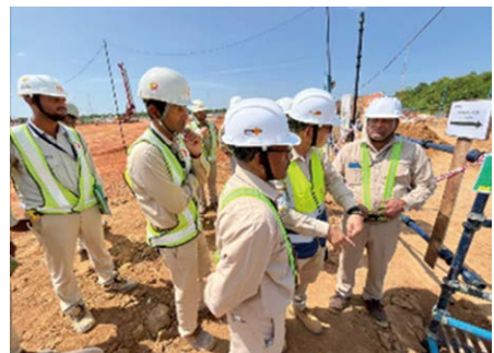
International PMS audit (on-site inspection)
