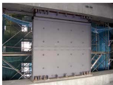
VDW Viscous Damping Wall
