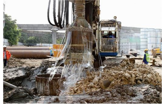
Fig. 2. Drilling of pile using polymer
