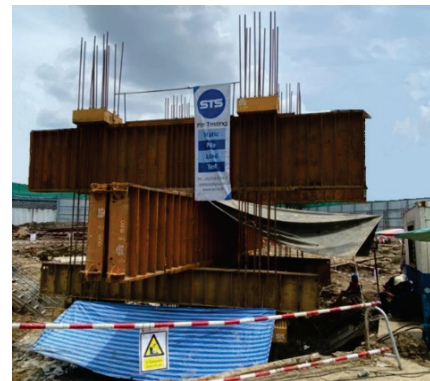
Fig. 4. Setting for static load test
