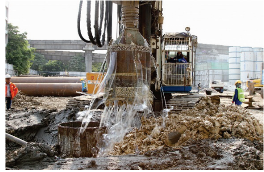
Fig. 2. Drilling of pile using polymer
