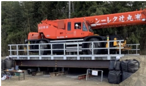
(c) Completed model bridge during load test
