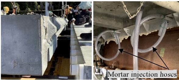
(a) Panel placement (b) Joint mortar injection
