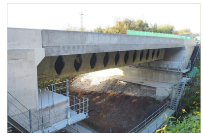
Fig. 2(c). Bessodani Bridge
