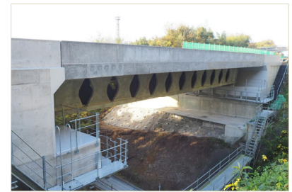
Fig. 2(c). Bessodani Bridge
