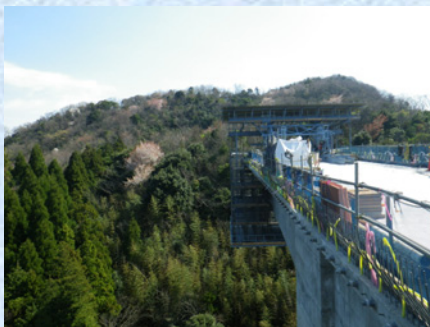
A1橋台部現況
