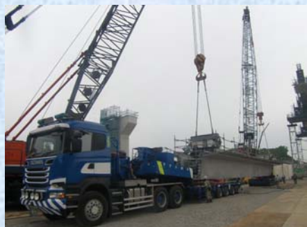
U桁積込運搬
